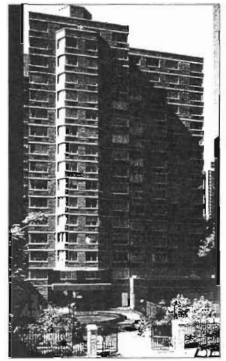
340 East 29th Street, Melzter/Mandl Architects
